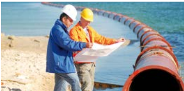
Floating in a ductile cast iron pipeline
