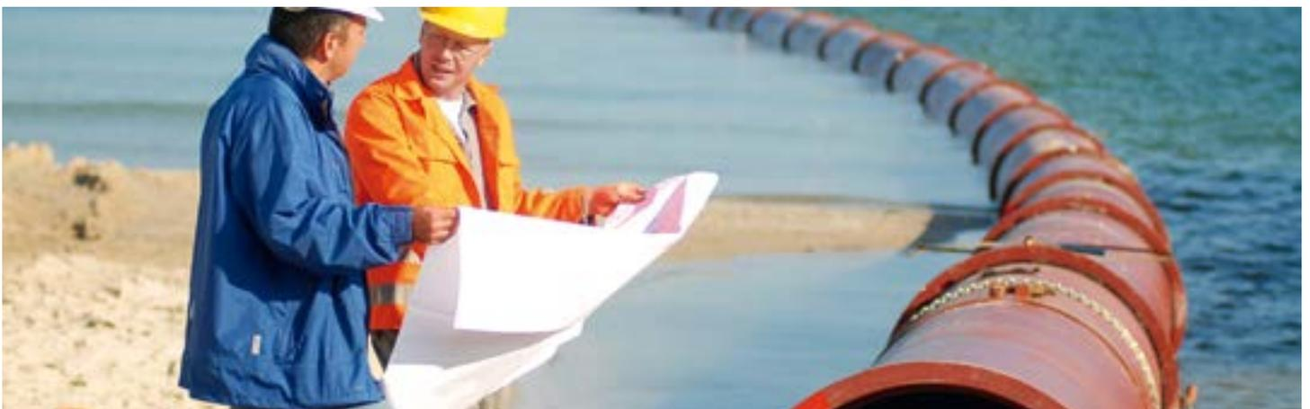
*Floating-in: the DN 1000 pipeline off Binz on the island of Rügen*
