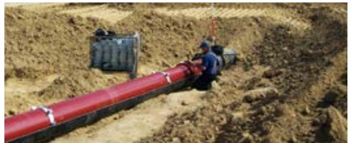
DN 400 ductile cast iron pipes with BLS®/VRS®-T socket joints being pushed into a stretch of protective tubes
