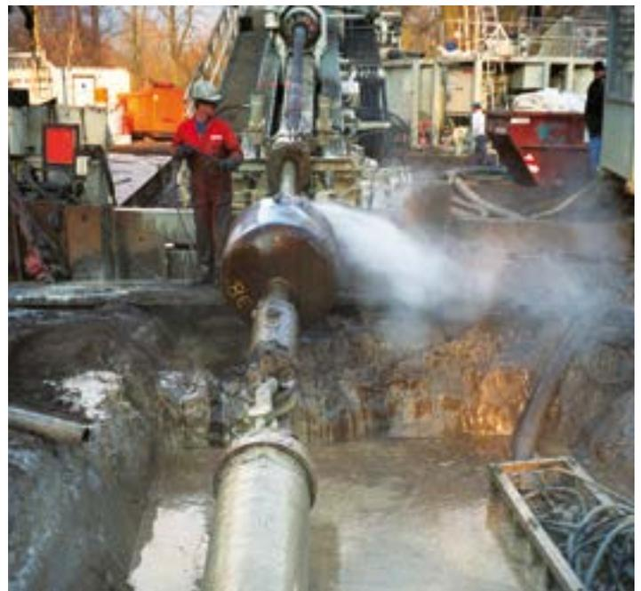
The horizontal directional drilling technique
